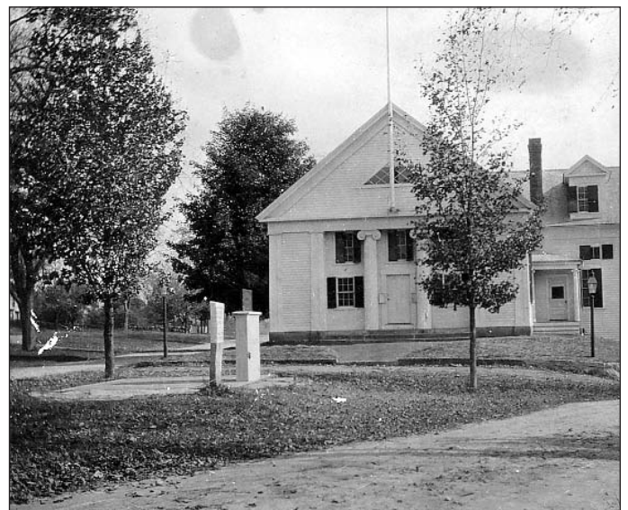
Hay was such an important crop in Stow that from 1870-1930 the town maintained an immense hay scale in front of Town Hall, where farmers could drive their loaded wagons directly onto it for weighing before taking their loads to market.
